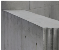
E - OFF-FORM CONCRETE CANDALEPAS ASSOCIATES - PERRY PARK
